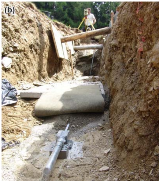
Fig. 2: (a) Schema of the strain rosette, (b) sensor S2 whilst embedding
