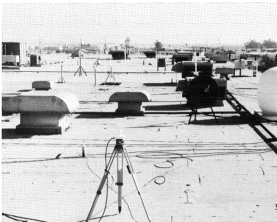
Figure 6: The roof of Building Three at the Magnavox plant in Torrance.
